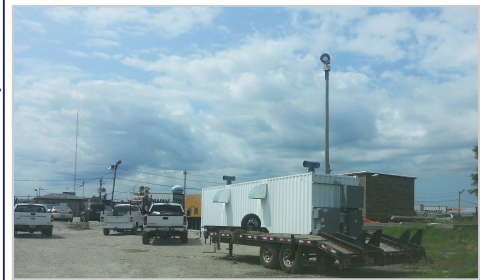
Well #3 Worksite near Roadway
